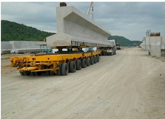
300 tonne concrete bridge section being trucked along a 400mm deep +10,000 Mpa RoadCem soil concrete road.
