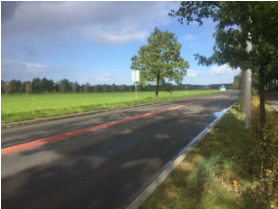
Figure 35 Asphalt on top of a RoadCem stabilization on Dutch road network, inspected by ARCADIS. No deformations occurred with standard axle load 100 kN.
